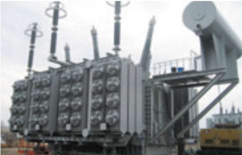
345kV Transformer
