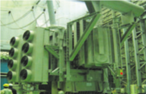
500kV Transformer
